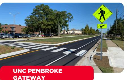
The main gateway to the UNC Pembroke campus in Robeson County was reconstructed in 2019, when NCDOT spent \$5 million overhauling a mile of North Odom Street/Prospect Road. A median, two roundabouts and sidewalks were built, making the roadway safer and more bicycle- and pedestrian-friendly. NCDOT proposed the design after university officials raised concerns over the safety of the students crossing it every day.
